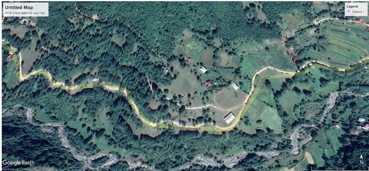
Pic. 3 Proposed route near village Khikhadziri, Khulo municipality (source-Google Earth Pro).
